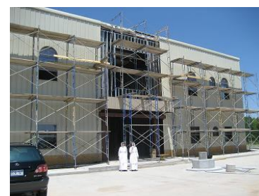
New Building of JVB HOUSTON
